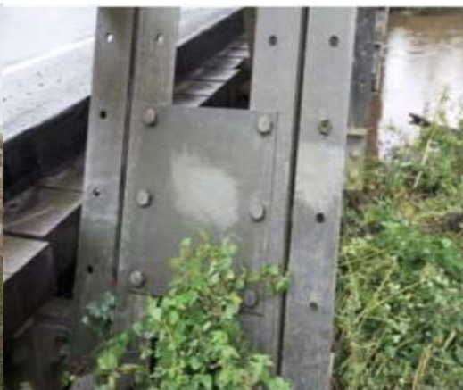
141.5 microns still offer for the C3 environment about 70 years of anticorrosive protection
